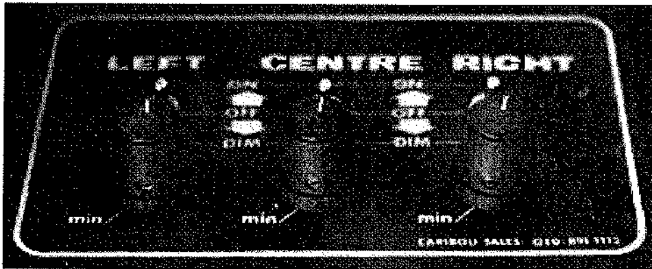
Figure 21. Lighting dimmer switches mounted on ceiling of Bell 412. courtesy of Westpac Rescue Helicopter base Broadmeadow.
